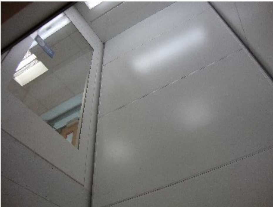
View going up in the lift looking at the floor above
