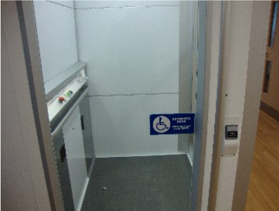
Front view looking into the lift from the landing
