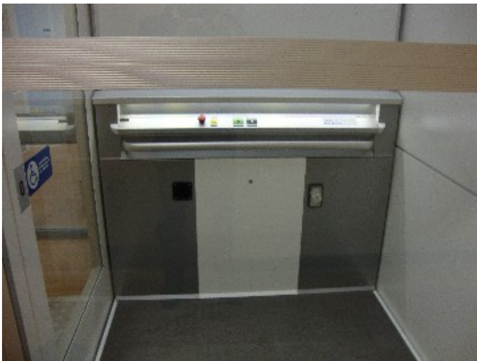
View looking through glass shaft to the platform
